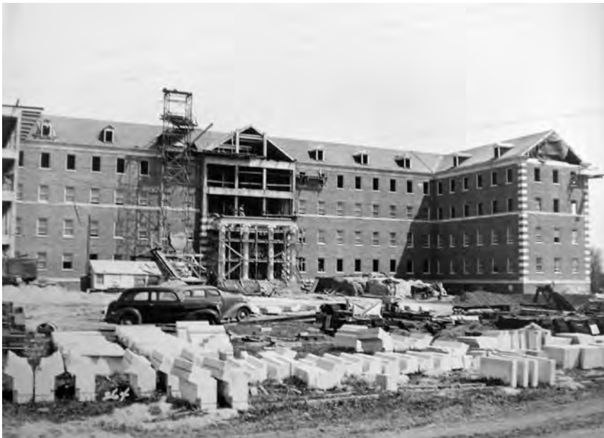
C. VA Building 9 nearing completion; (PWA, ca. 1943)
