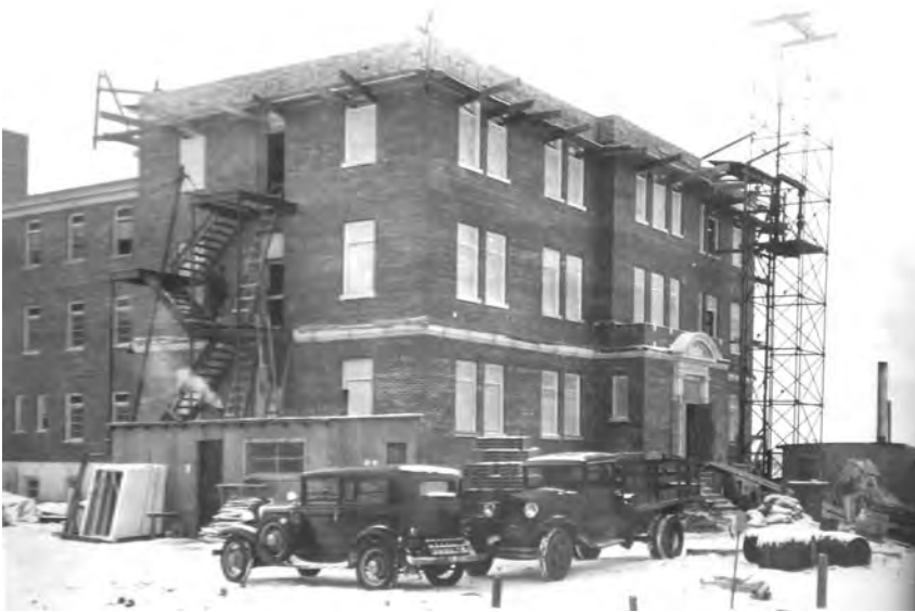
A. Addition to VA Building 1 infirmary, under construction, (PWA 1934)
