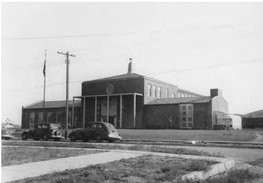
Fig. 21: Historic photos of jobsite work conditions; top : Dormitory construction at Grafton State School for the Feebleminded (1936), and lower : Sunnyside Grade School, Minot, ND (1938-39) Selected images reproduced from papers and records of Edwin W. Molander, reproduced courtesy of the State Historical Society of North Dakota, State Historic Preservation Office
