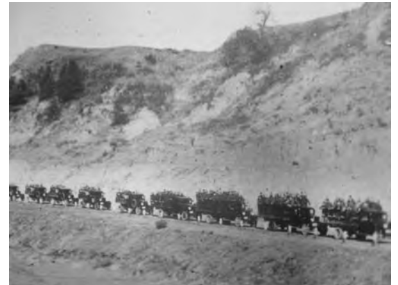
B. CCC company being transported locally by construction work trucks, from Medora train station and camp sites to project sites
