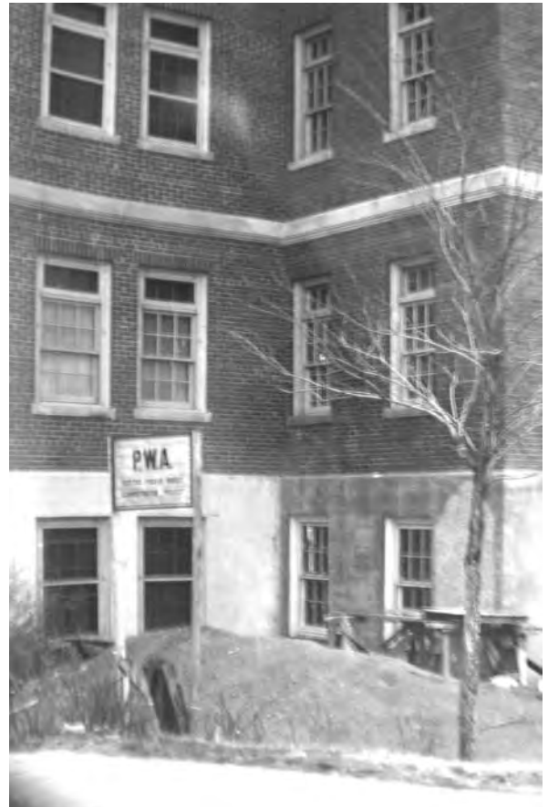
B. VA Building 1 infirmary under construction; note PWA project office on-site, (1934).
