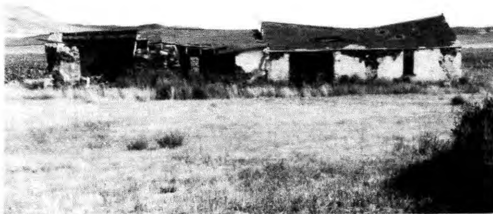
Figure 18. Exposed ridgebeam is visible at left. Jacob Brittner Farmstead [SK 32 188].
