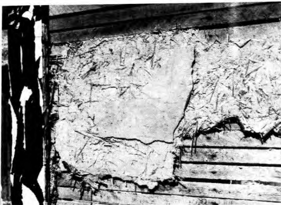
Figure 24. Clay/straw/manure plaster on interior lath. George Weiler House [32 SK 157].
