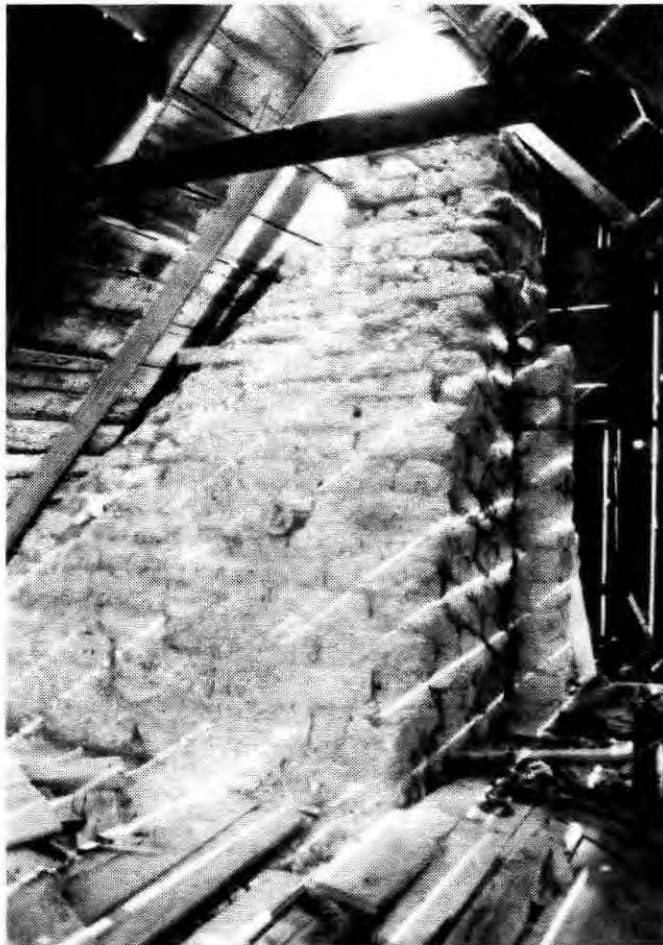
Figure 43. Detail of mud brick flue. Smokehouse at Martin Farmstead [32 SK 189].
