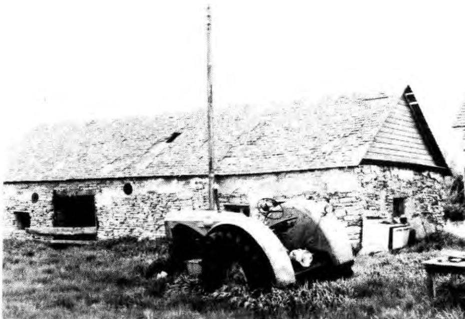
Figure 39. Original one-room house (right) and barn addition (left) at the Frank/Vogel Farmstead [32 SK 158].
