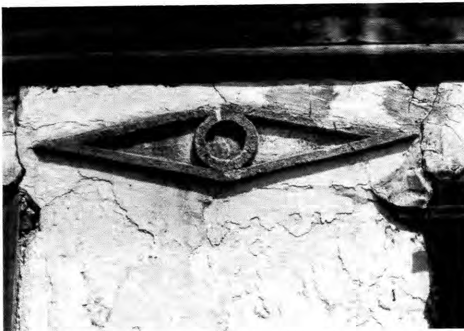
Figure 23. Detail of raised stucco ornamentation at the John Reiner House [32 SK 159].
