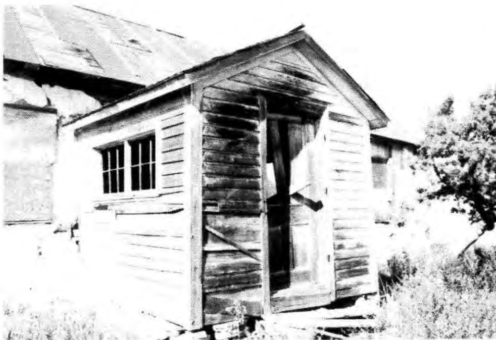
Figure 19. Detail of wood frame "vorhausl" on the Philip Loran house [32 SK 190].
