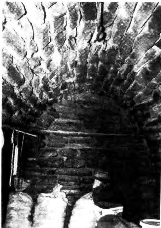
Figure 45. Detail of root cellar at R. Frank Homestead [32 SK 156].
