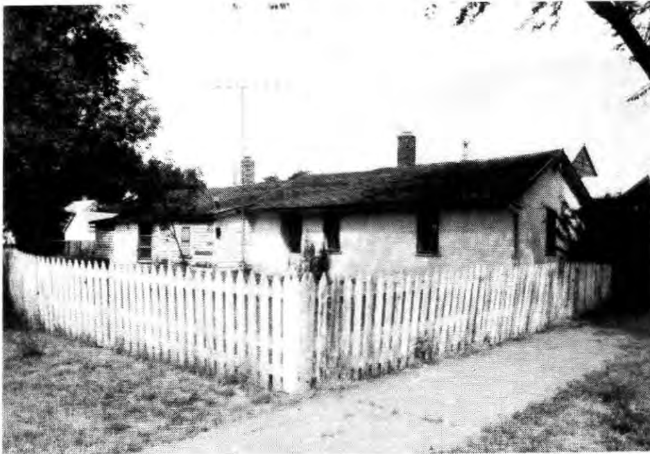
Figure 48. The Urlacher House [32 SK 198] in south Dickinson. This is a stone house with a wood frame addition.
