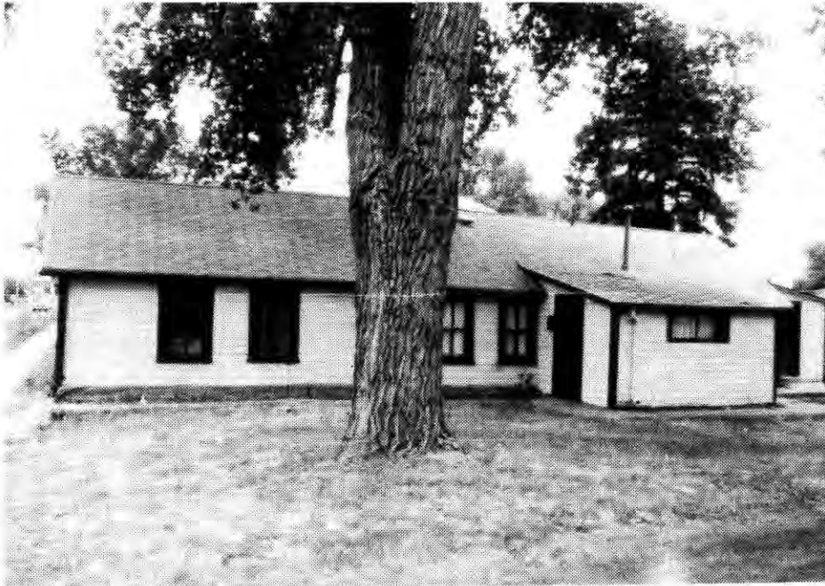
Figure 49. The Schoch House in south Dickinson. This house is constructed of vertical railroad ties, covered with drop siding.
