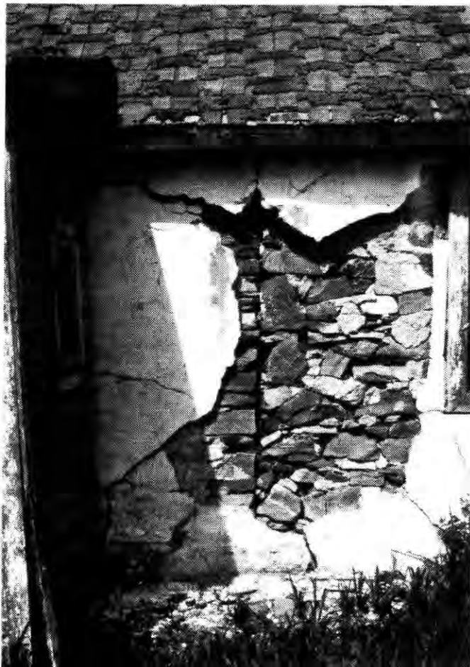
Figure 17. Evidence of addition to the Mathias Link House [32 SK 155].
