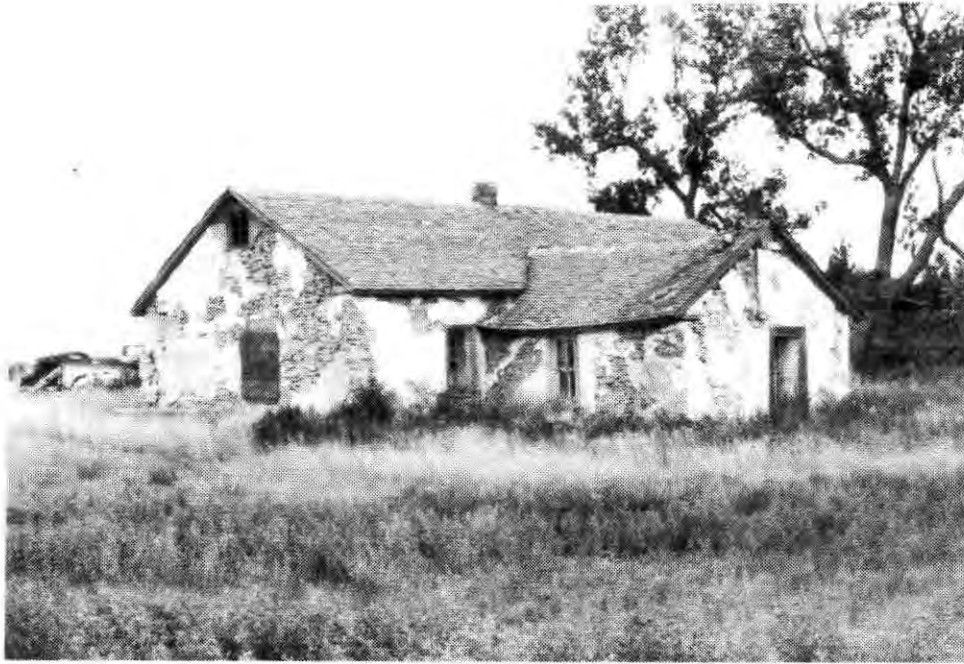
Figure 27. Berger House [32 SK 164] showing large kitchen addition to the facade.
