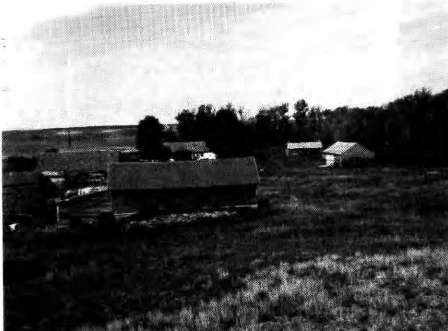
Figure 12. Courtyard arrangement of buildings at the Mathias Link Farmstead [32 SK 155].
