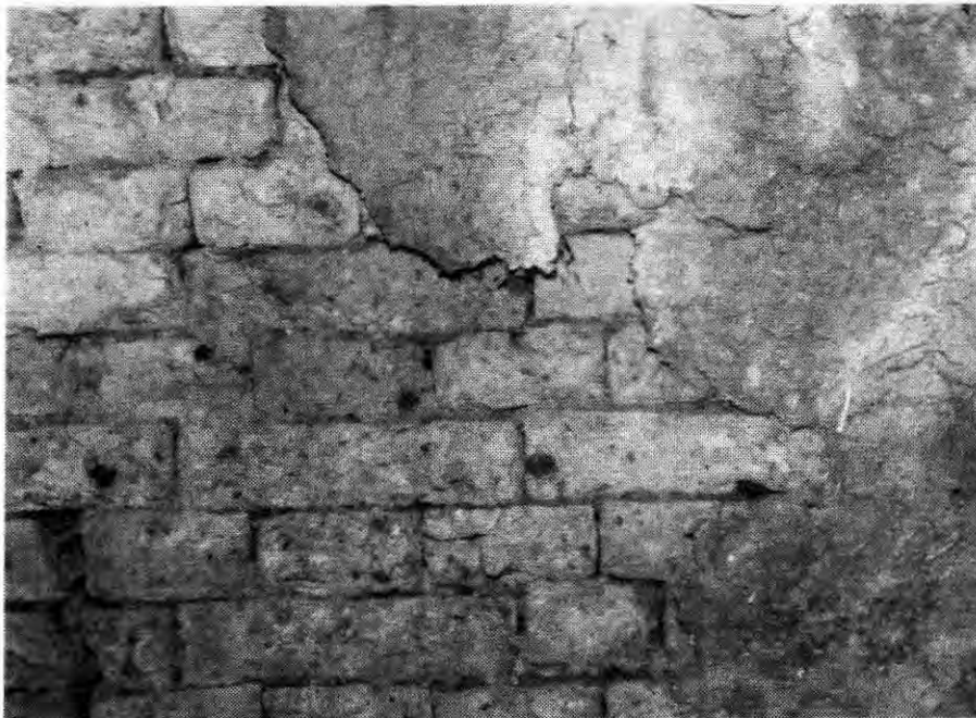
Figure 32. Detail of mud brick wall. Schneider House [32 SK 173].
