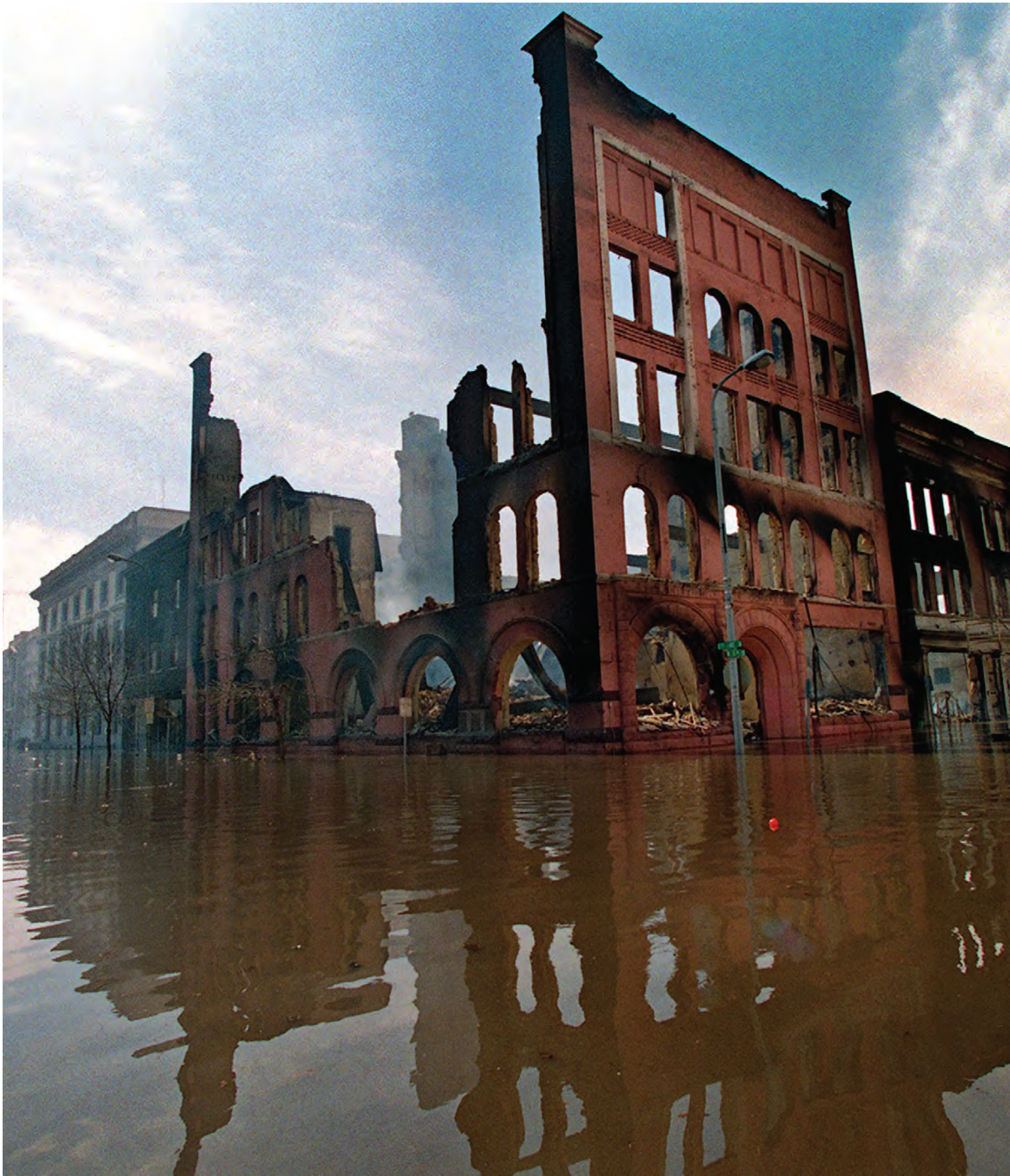
The Security Building, the first of eleven downtown Grand Forks buildings to go up in flames, stands in ruins on April 20, 1997. Eric Hylden/Grand Forks Herald, April 21, 1997
