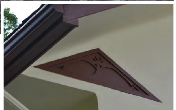
Unlike the patterned shingles or lace-like spindle work of Victorian-era Queen Anne houses or the fluted columns and ornate cornices of contemporary Classical revivals, exterior ornament found on Prairie Style residences is typically restrained, often intended to emphasize the horizontality of the structure. Examples include the use of contrasting trim between stories and recessing horizontal masonry joints in brickwork. The P. E. Byrne house exhibits both of these techniques and boasts the added charm of wood-carved eave details with a flora motif inspired by natural forms. Photo by author
