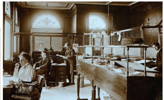
Interior of Bismarck's First National Bank prior to the 1912 renovation. Second and third from left are bank employees Leonard Bell and Dick Peuwarden. SHSND SA 2004-P-023-00004
